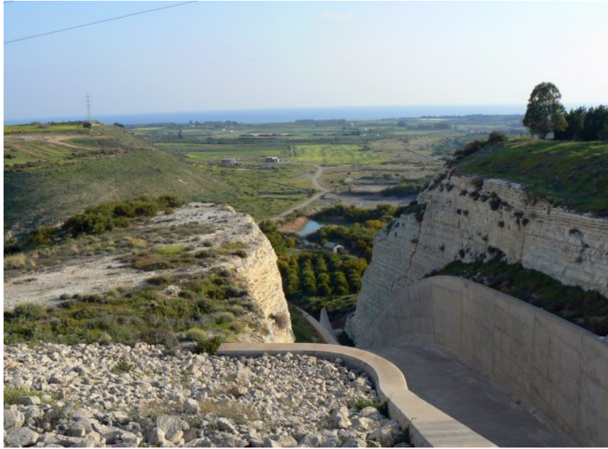
Asprokremnos Dam pools from the dam
